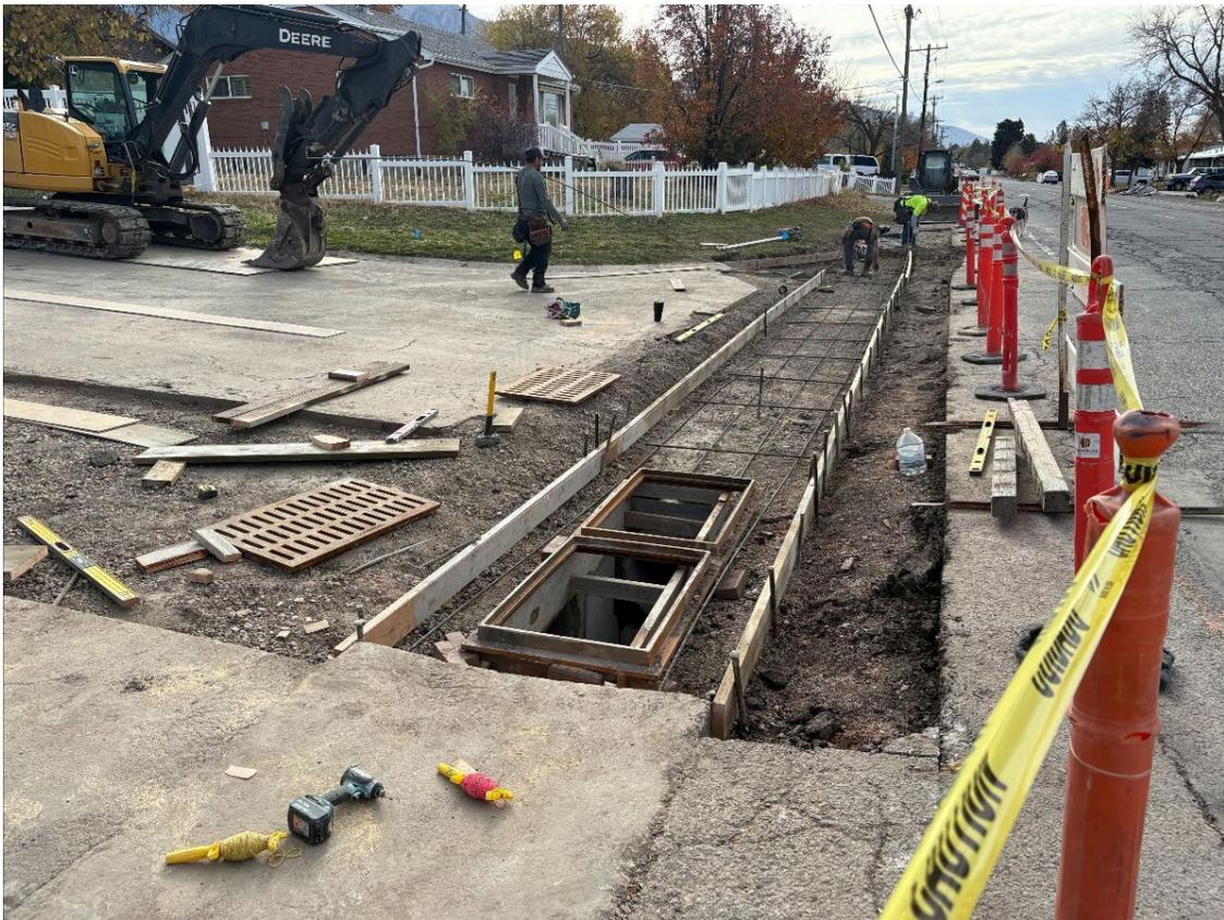
**THE SOLUTION - new storm drain inlets and waterway shown during construction**
